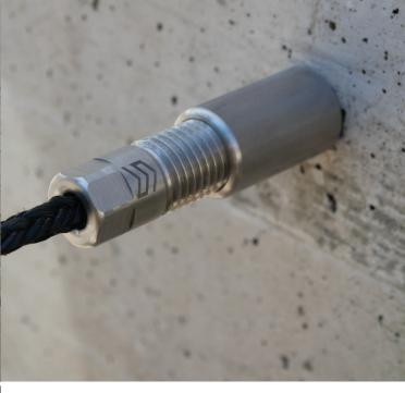
Adhesive anchors are casted or post-installed into concrete parts.
